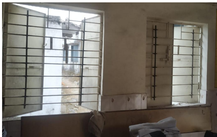
06 windows were repaired with tightening the gap with extra rod for more protection
