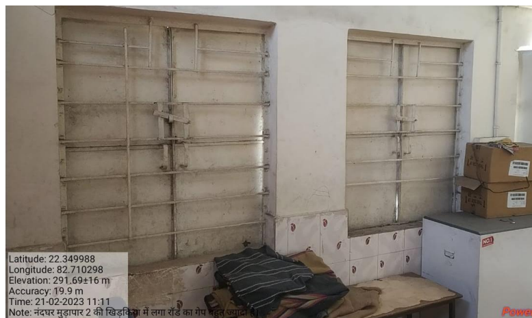
06 windows were repaired with tightening the gap with extra rod for more protection
